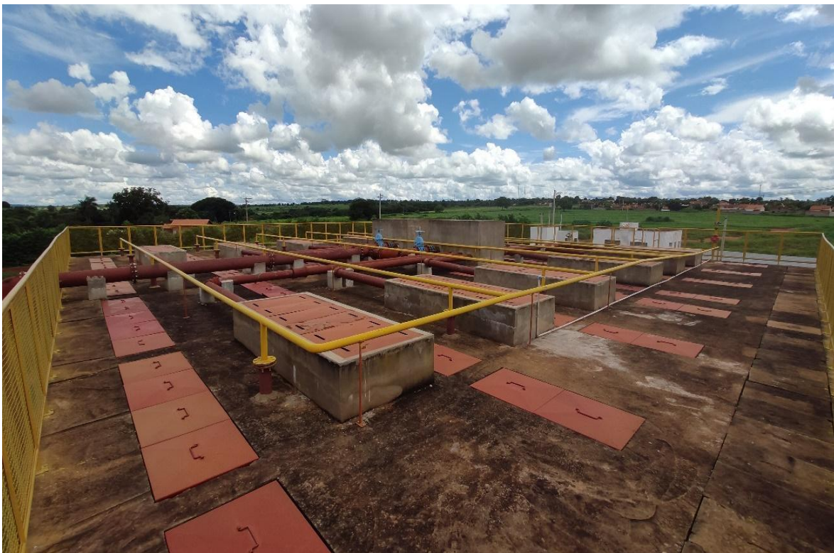
Figura 118: Reator UASB
